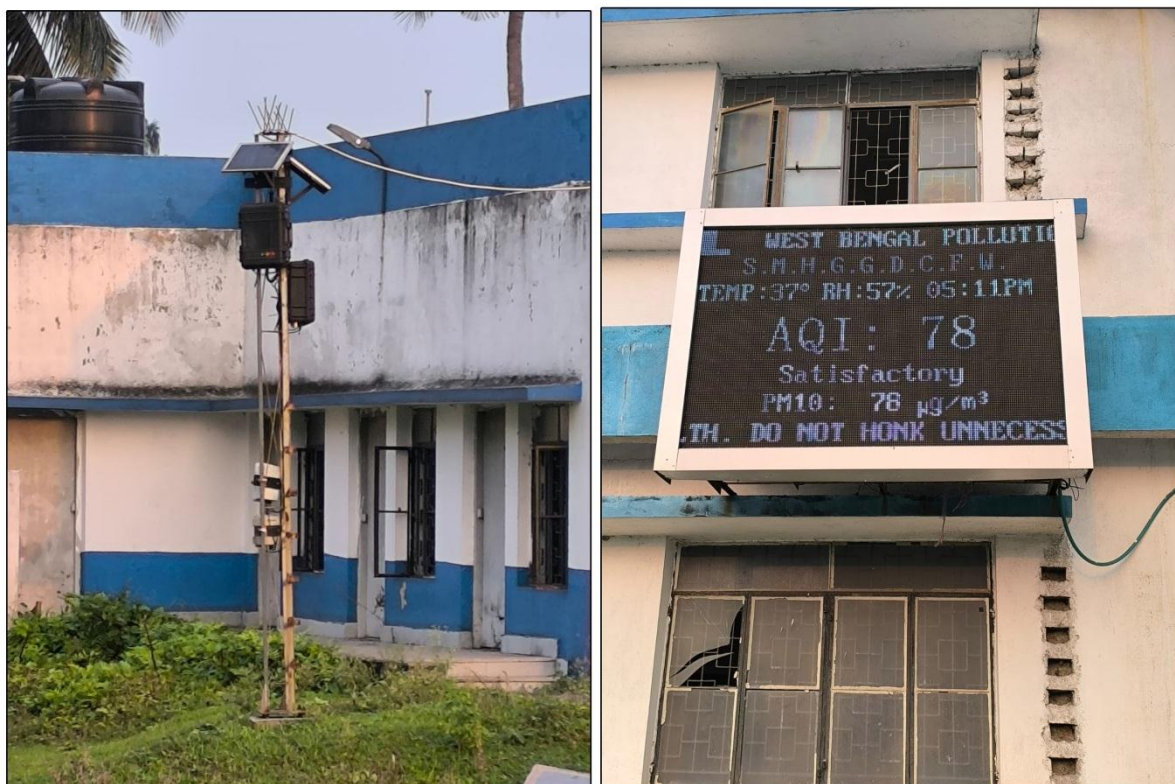
Plate 1: WBPCB Air Quality Monitoring Station at Shahid Matangini Hazra Government General Degree College for Women. Left: Monitoring station; Right: Display board
